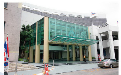
PTT PUBLIC COMPANY LIMITED ; RENOVATION
