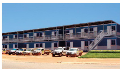
AUSTRALIA ; FMG PROJECT 720 MAN CAMP
